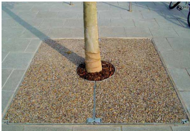
NEAT FINISHES WHICH ARE ACCESSIBLE FOR MAINTENANCE
