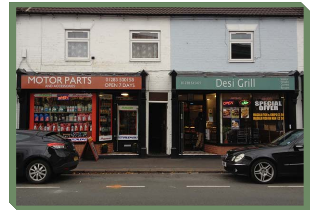
AFTER: BY FOLLOWING A NUMBER OF BASIC PRINCIPLES AND INCLUDING TRADITIONAL ELEMENTS IN THE DESIGN OF SHOP FRONTS, THESE ISSUES ARE OVERCOME.
