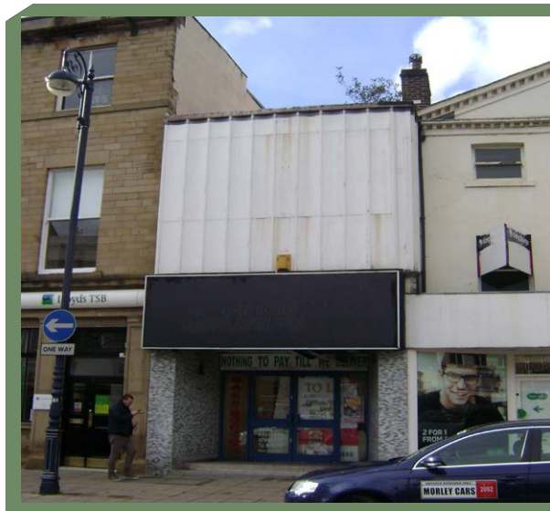
INAPPROPRIATE ALTERATION ON A PRIMARY FRONTAGE
