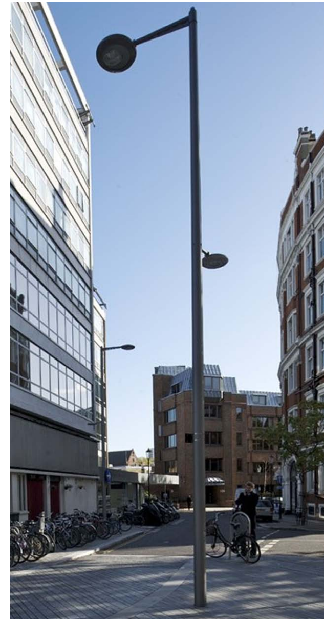
TO PROVIDE FUNCTIONAL LIGHTING WHICH ACCOMMODATES VARYING USERS WHILST REDUCING STREET CLUTTER
