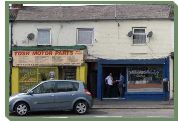
BEFORE: LACK OF TRADITIONAL ELEMENTS CREATES A LOSS OF RHYTHM. THERE IS NO RELATIONSHIP BETWEEN THE SHOP AND UPPER FLOORS.
