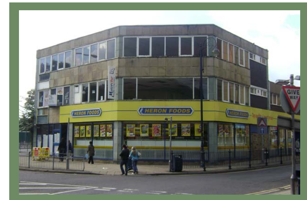
INAPPROPRIATE FORM AND HORIZONTAL EMPHASIS
