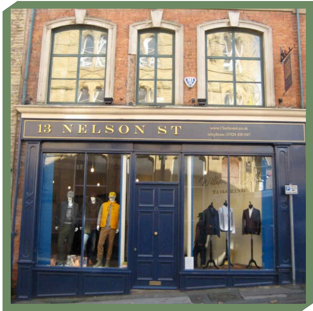
GOOD EXAMPLE OF A PERIOD SHOP FRONT, DEWSBURY
