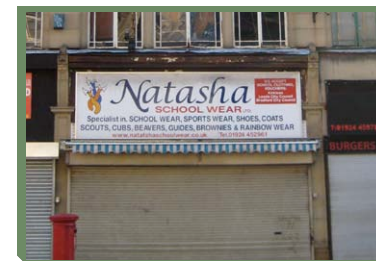
EXTERNALLY MOUNTED SHUTTERS CREATE A HOSTILE ENVIRONMENT AND SHOULD BE AVOIDED
