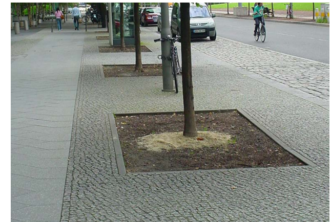
PROVIDE ADEQUATE SPACE FOR TREE PLANTING IN ORDER TO ENSURE HEALTHY GROWTH
