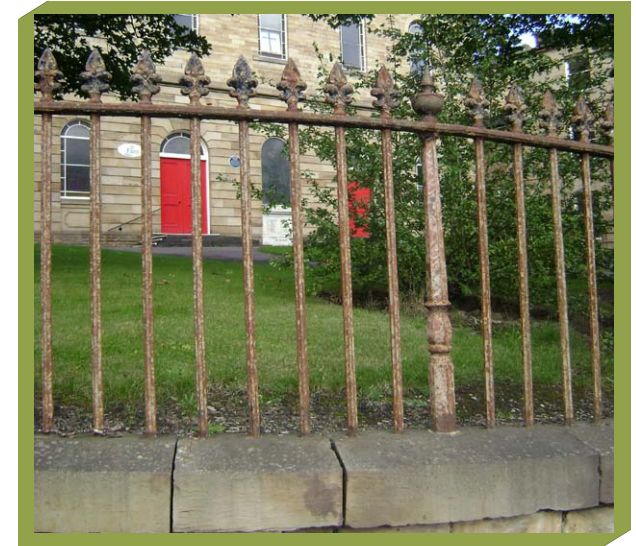
PROVIDE ADEQUATE SPACE FOR TREE PLANTING IN ORDER TO ENSURE HEALTHY GROWTH
