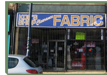
EXTERNALLY MOUNTED SHUTTERS WITH SEE THROUGH MESH AND INTEGRATED INTO THE FACIA ALLOW VIEWS INTO THE SHOP.
