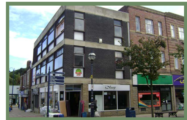
INAPPROPRIATE DETAILING AND MATERIALS
